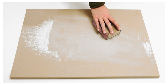
4. To partially restore the surface, use the wooden block (D) with the sandpaper P240 (B).
