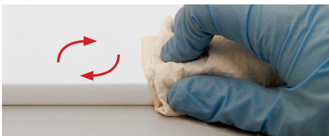
9. Rub up vigorously with polish (I) to give the surface its initial shine.
