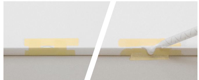
6. Cover the area to be repaired with a plentiful layer of product. Let it dry for 2 hours at a minimum temperature of 15/18°C. Do not wet the surface.
