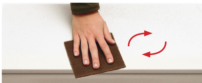
9. Wipe a Scotch-Brite pad (D) in the direction shown above until the surface is completely smooth.
